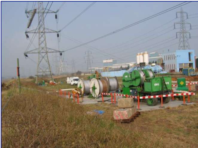
Photograph 4.4a and 4.4b – Machinery Associated with Conductor Pulling on Trackway
