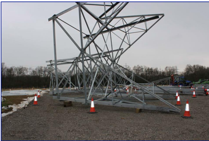
Photograph 4.2a – Steelwork Preparation on the Ground; and 4.2b – Pylon Erection
