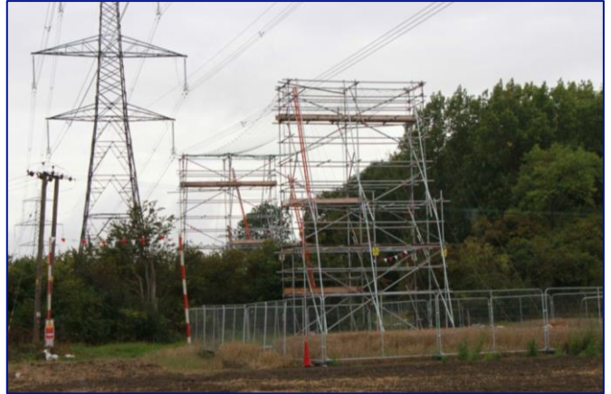
Photograph 4.3a – Scaffold Protecting a Road; and 4.3b – Protecting an 11kV Pole Line
