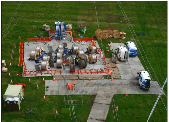
Photograph 4.4a and 4.4b – Machinery Associated with Conductor Pulling on Trackway
