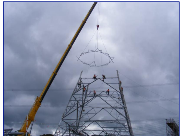
Photograph 4.2a – Steelwork Preparation on the Ground; and 4.2b – Pylon Erection
