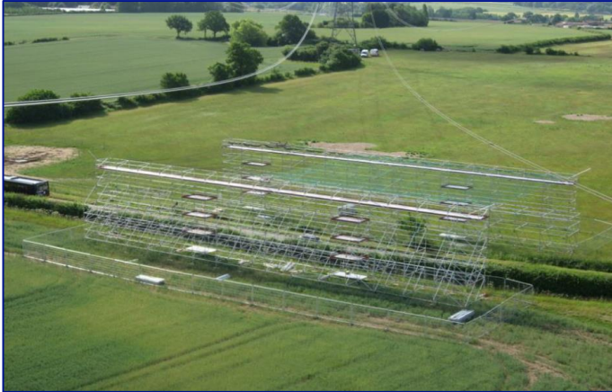
Photograph 4.3a – Scaffold Protecting a Road; and 4.3b – Protecting an 11kV Pole Line
